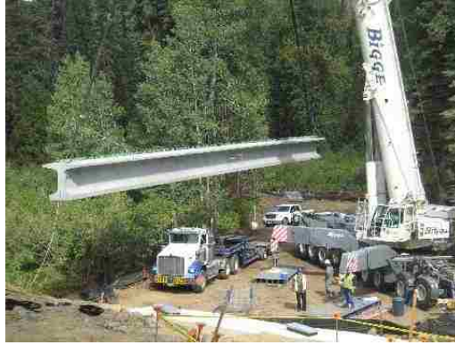
Figure 1.1. A precast DBT girder being lifted into place by a crane.
