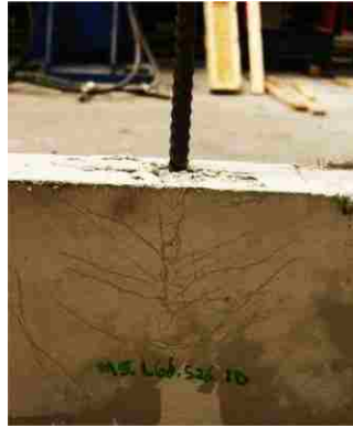
Figure 7.5. Diagonal crack pattern observed by Graybeal.
